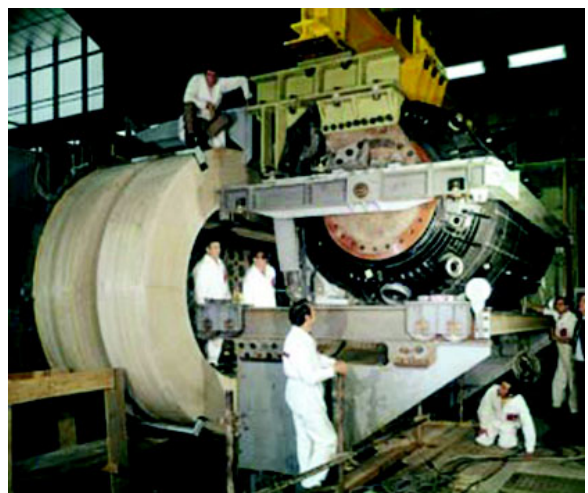
Fig. 1: The Gargamelle heavy-liquid bubble chamber, installed into the magnet coils, at CERN in 1970.
